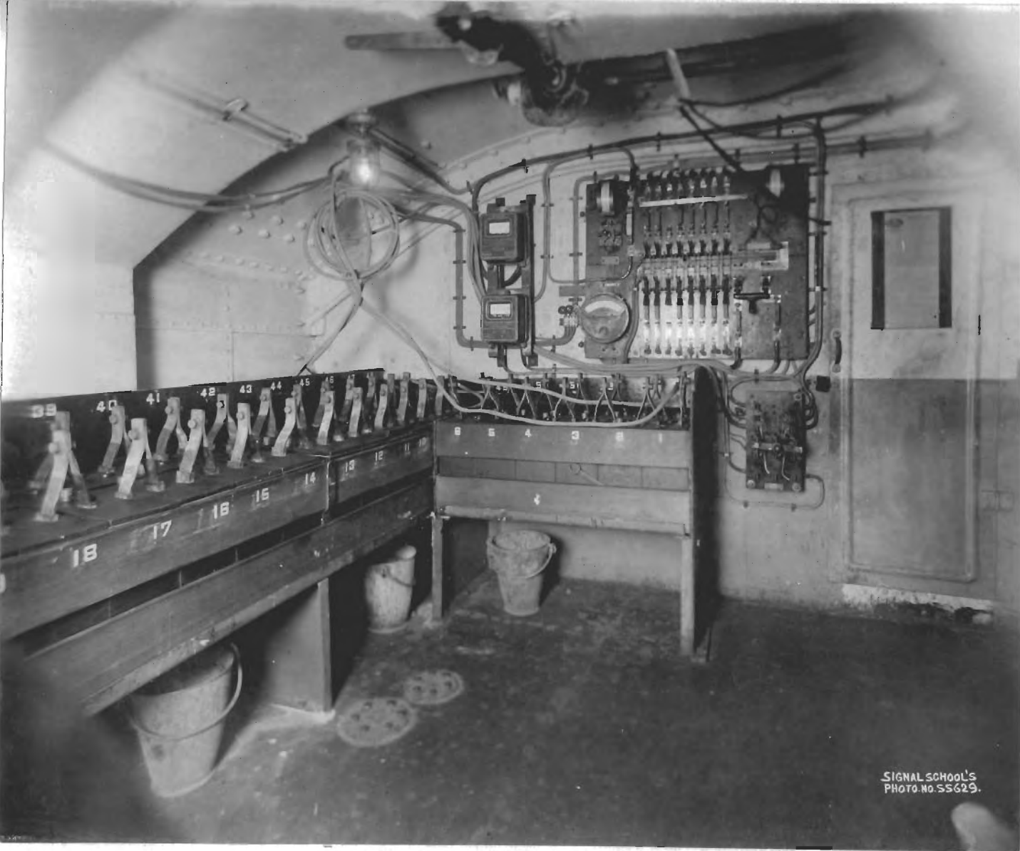
Fig. 21. BATTERY ROOM IN H.M.S. "AGAMEMNON"
