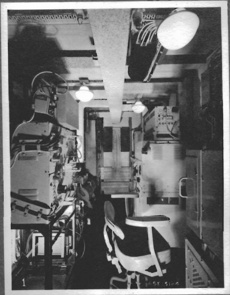
No.1 INTERIOR OF LOWER HALF.
